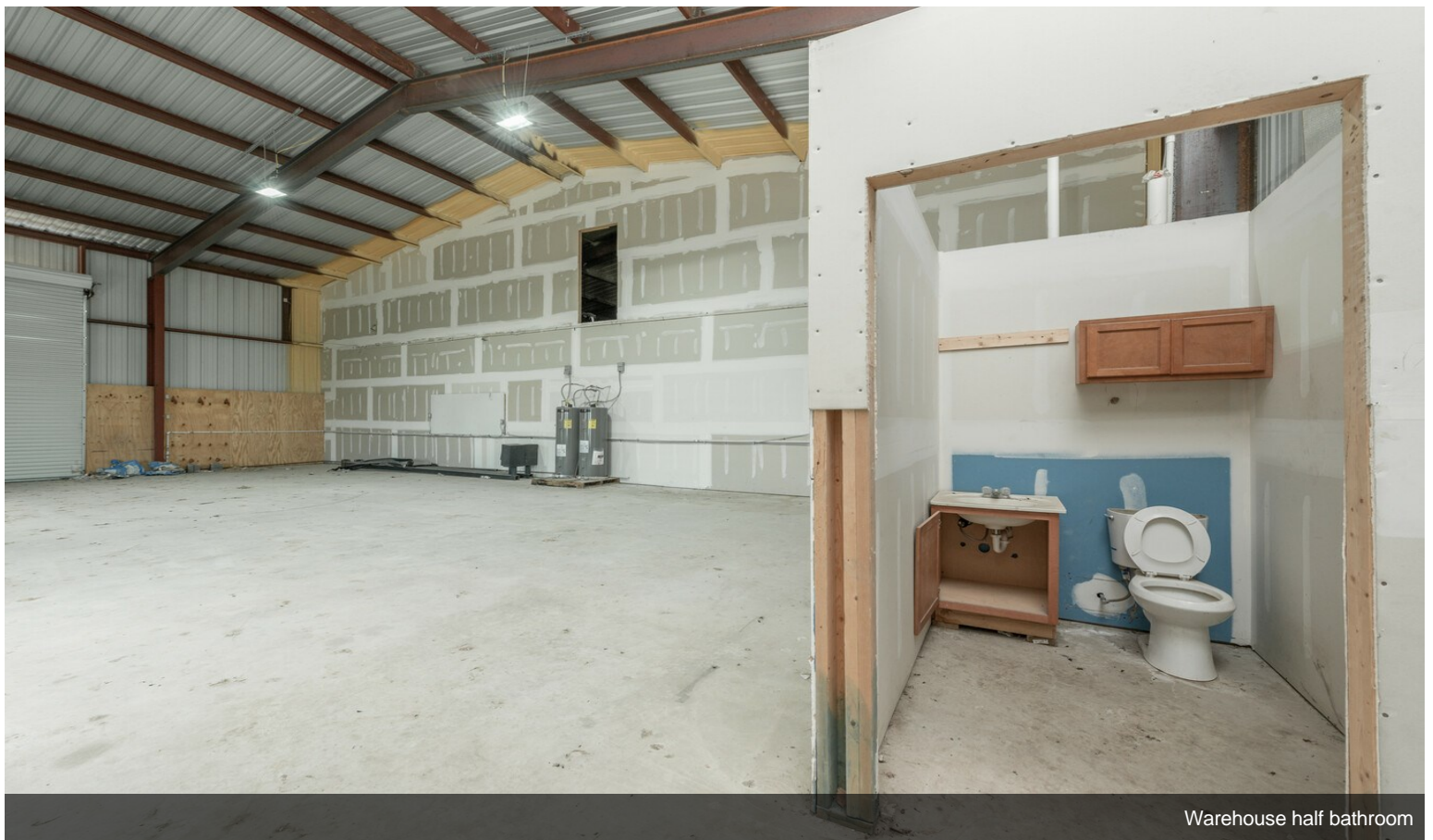
Warehouse view from 14' Bay
