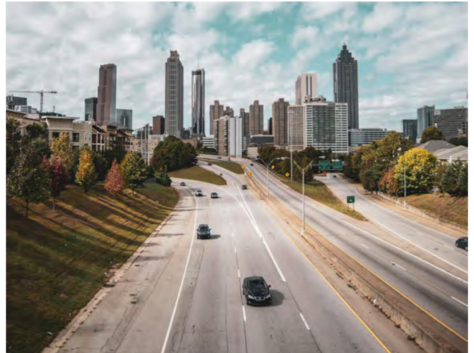
Jackson Street Bridge, Atlanta
