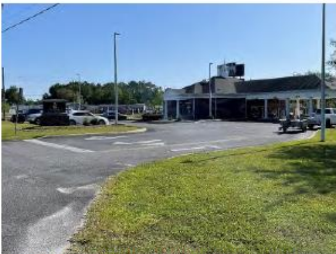
WEST EXTERIOR AND PARKING AREA
