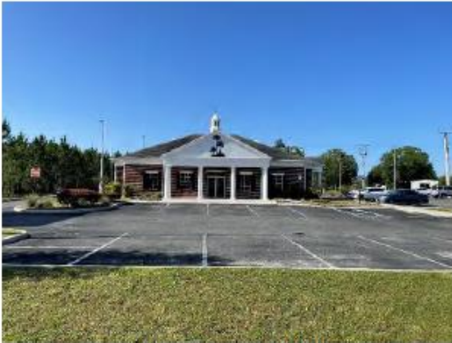
NORTH EXTERIOR AND PARKING AREA
