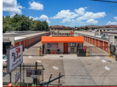
All Storage of Elk Grove
