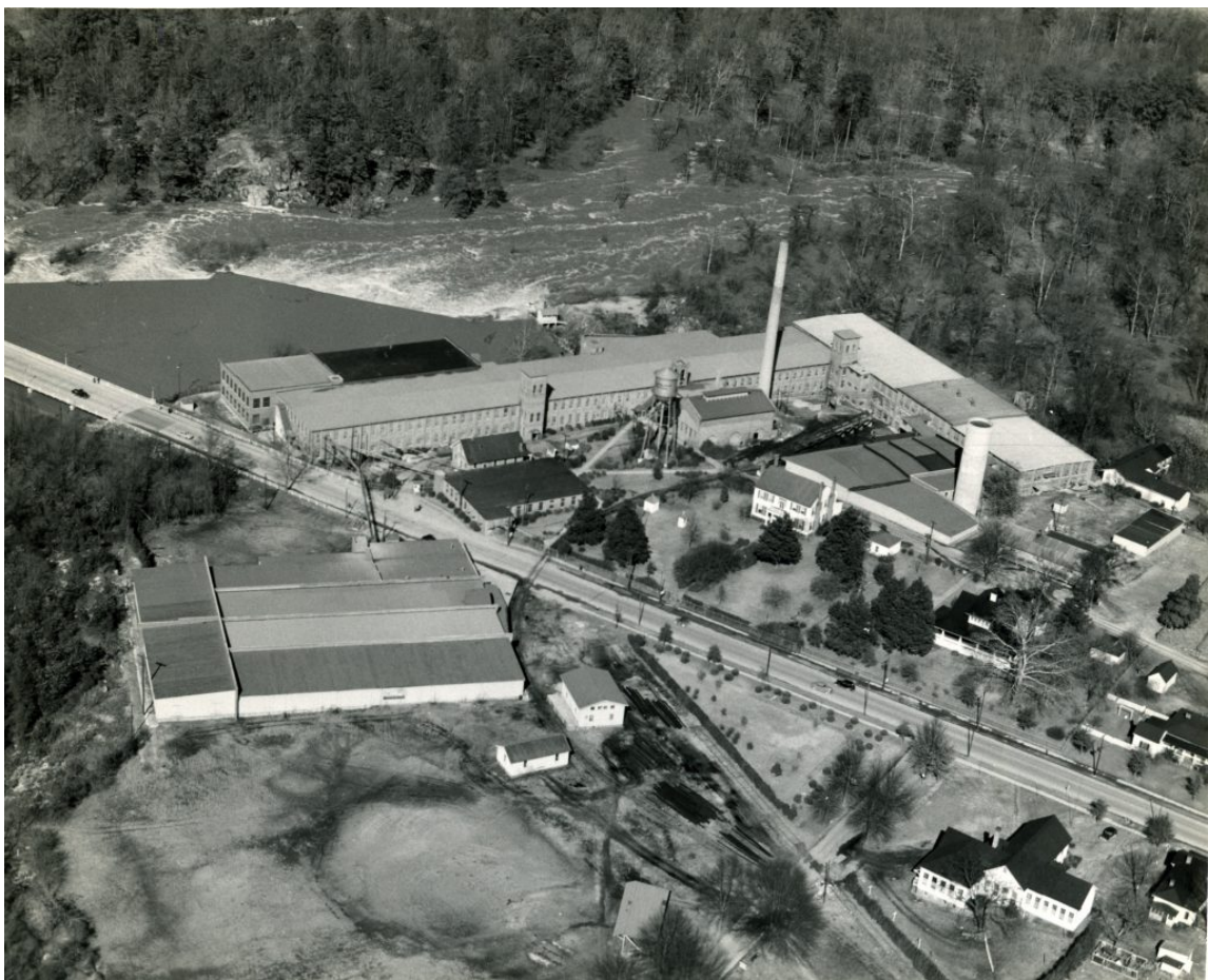
An old aerial shot of the mill. Source: Rocky Mount Mills.
