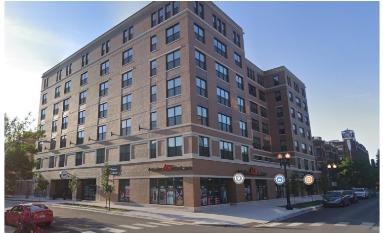
Southeast Corner of Sheridan and Dakin—New construction Loft building with tenants Ace Hardware and Artemio's Bakery
