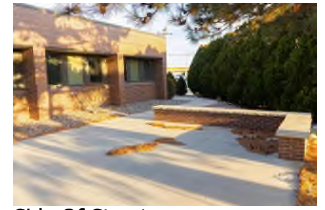
Side Of Structure
