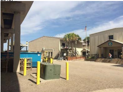
View of Building 3, Looking North (Photo Taken on November 1, 2018)
