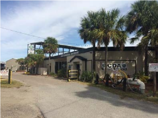
Front View of Building 1, Looking North (Photo Taken on November 1, 2018)
