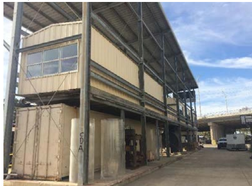
View of Building 4, Looking Southwest (Photo Taken on November 1, 2018)
