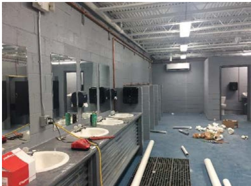
View of Building 2 Restroom/Shower (Photo Taken on November 1, 2018)
