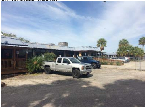
View of Building 6, Looking Northwest (Photo Taken on November 1, 2018)
