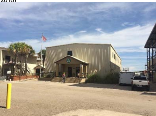
View of Building 5, Looking Northeast (Photo Taken on November 1, 2018)
