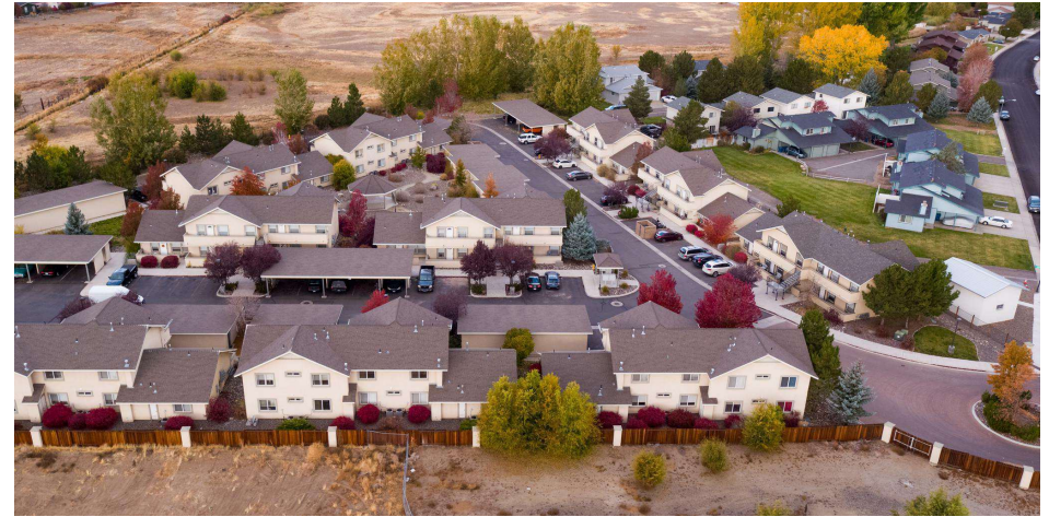
1 Pebble Creek Apartments 1454 Hussman Ave Gardnerville, NV 89410
