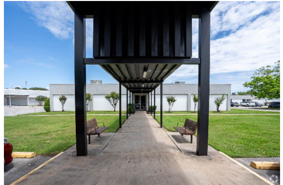
1600 - 1610 Connecting Canopied Walkway
