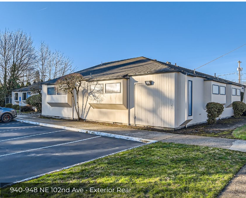
940-948 NE 102nd Ave - Exterior Front
