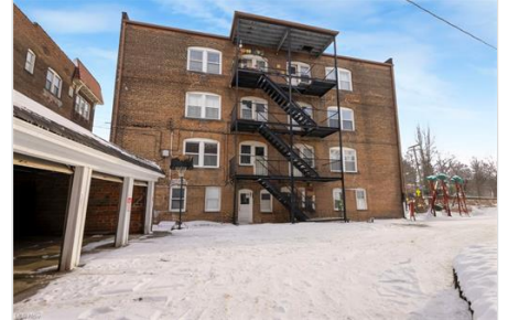
Back of Structure
