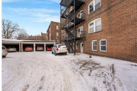
Back of Structure
