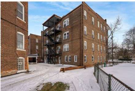
Back of Structure
