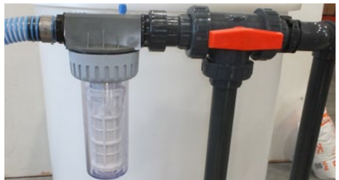
Heavy duty filter and 3-way valve
