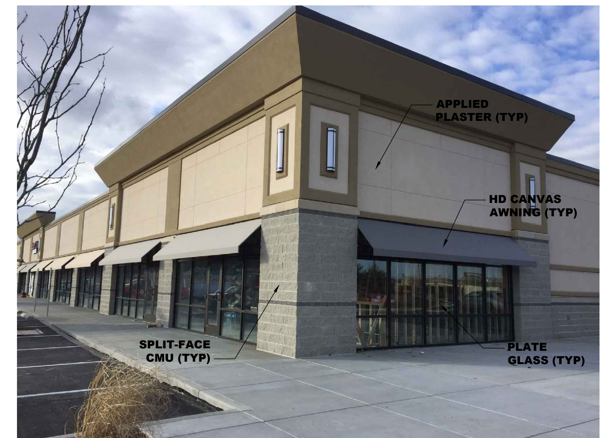
RETAIL BUILDING ELEVATION "B" NTS
