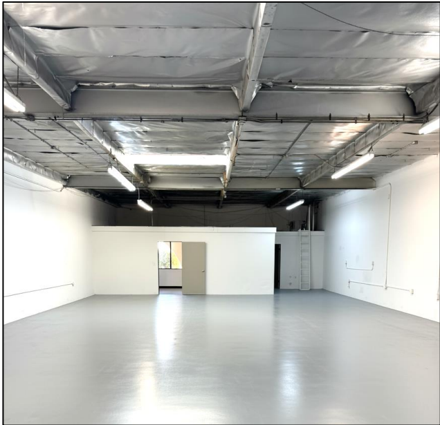
Warehouse facing forward with Office and Skylight
