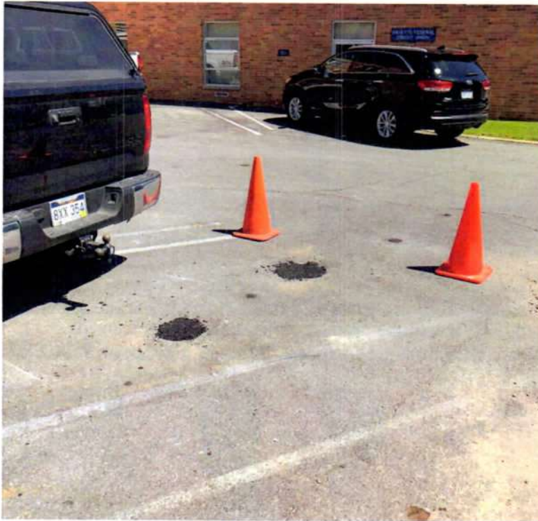
View of the UST ports filled with asphalt patch. Photo taken from the southwest, facing northeast, on 9/4/2018.
