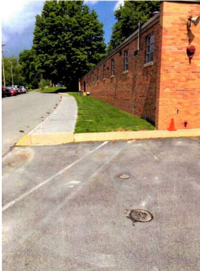
View of the tank 1,000-gallon #2 fuel oil UST location. Photo taken from the southeast, facing northwest.
