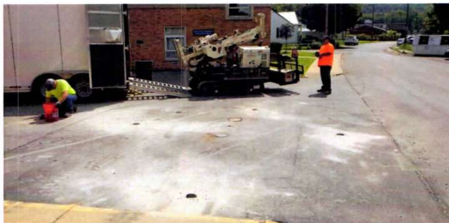
View of East Wall, North Wall, South Wall, and West Wall soil boring locations. Photo taken from the northwest, facing southeast, on 8/15/2018.
