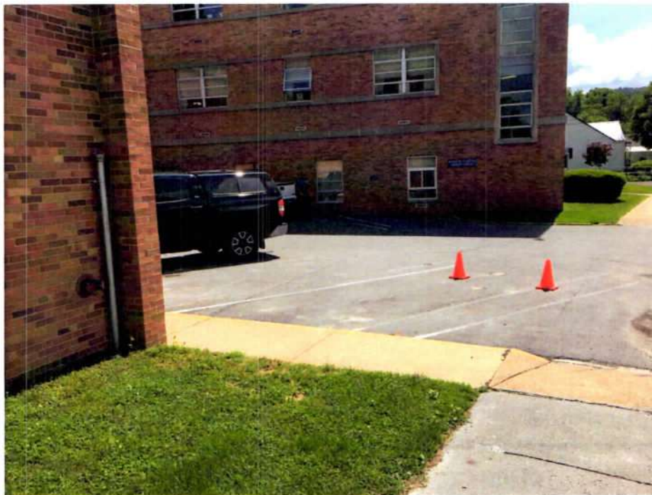
View of the tank 1,000-gallon #2 fuel oil UST location. Photo taken from the west, facing east, on 8/14/2018.
