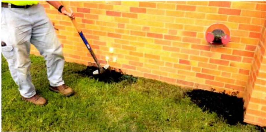
View of the product piping area, reclaimed. Photo taken from the south, facing northwest, on 9/20/2018.
