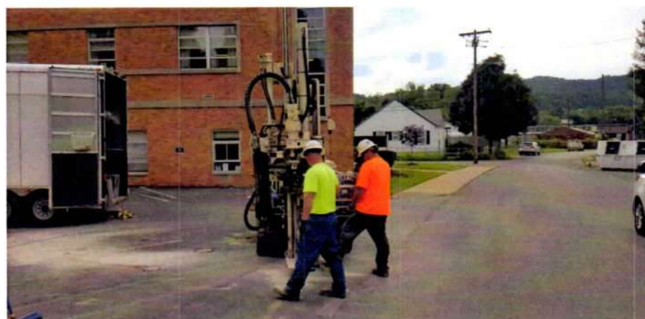
View of the drill crew working on the south wall of the tank. Photo taken from the west, facing east, on 8/15/2018.
