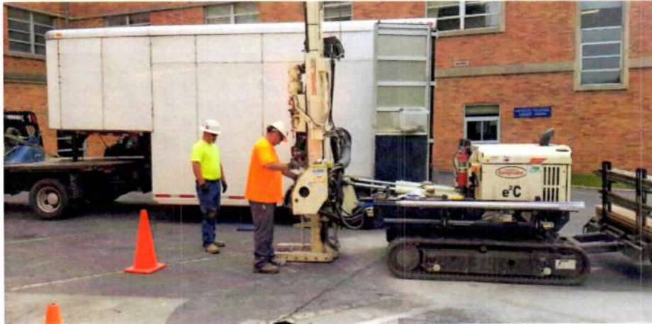
View of the drill crew working on the east wall of the tank. Photo taken from the west, facing east, on 8/15/2018.
