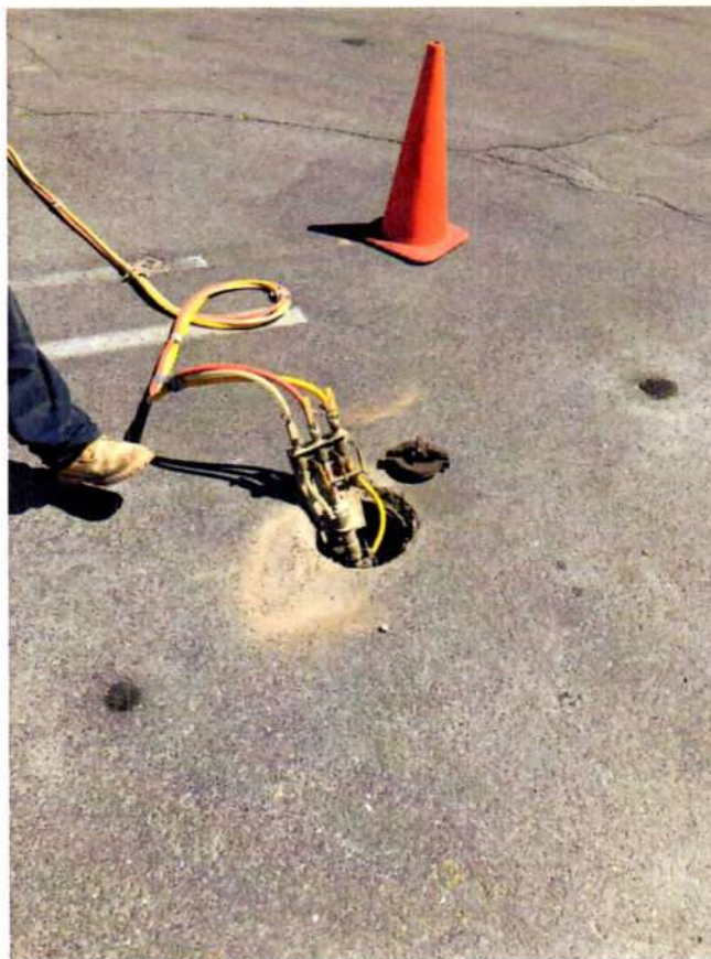
View of the foam filling process. Photo taken from the southwest, facing northeast, on 9/4/2018.
