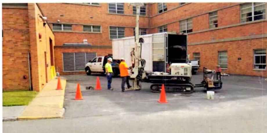
View of the drill crew working on the north wall of the tank. Photo taken from the southwest, facing northeast, on 8/15/2018.
