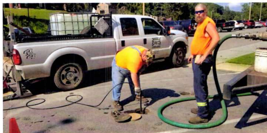
View of the Envirocheck crew cleaning the inside of the UST. Photo taken from the northeast, facing southwest, on 8/14/2018.
