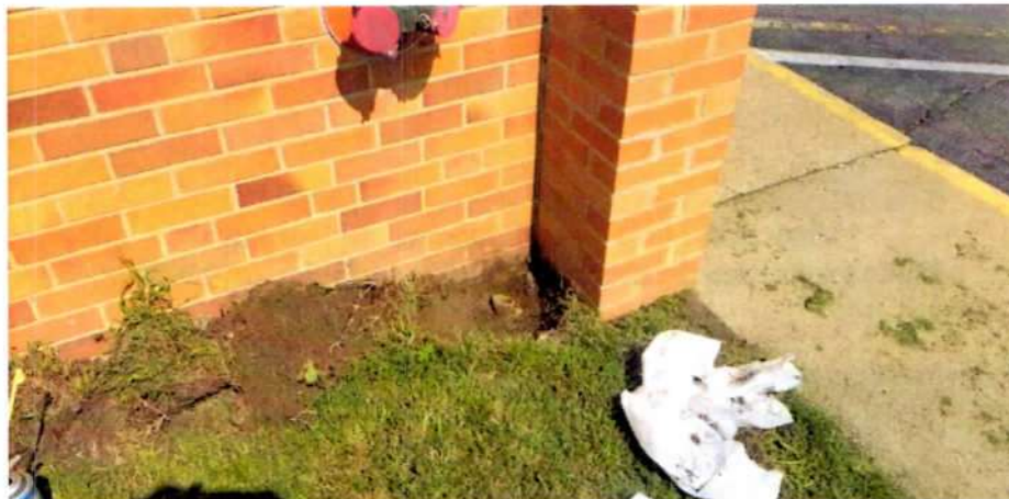
View of the vent pipe, removed. Photo taken from the southwest, facing northeast, on 9/20/2018.
