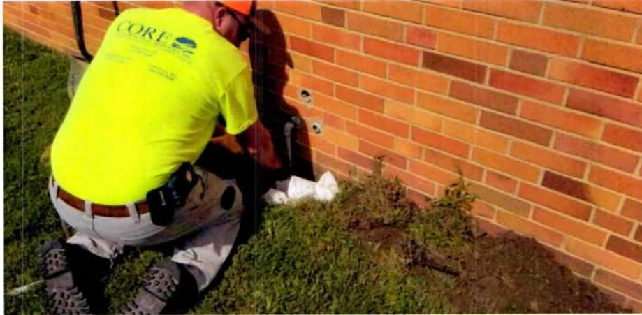
View of the product piping being disconnected. Photo taken from the southeast, facing northwest, on 9/20/2018.
