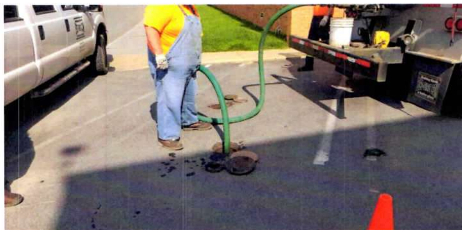
View of Envirocheck crew removing fuel from UST. Photo taken from the east, facing west, on 8/14/2018.
