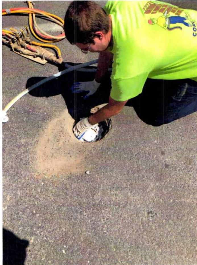
View of the crew filling the 1,000-gallon tank with foam. Photo taken from the southwest, facing northeast, on 9/4/2018.
