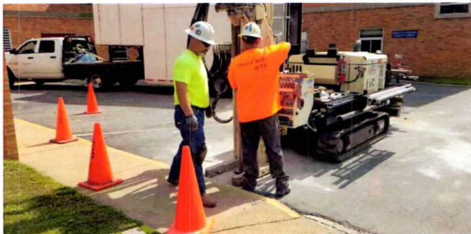
View of the drill crew working on the west wall of the tank. Photo taken from the southwest, facing northeast, on 8/14/2018.
