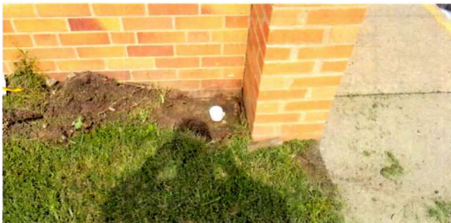
View of vent pipe, capped. Taken from the south, facing northeast, on 9/20/2018.
