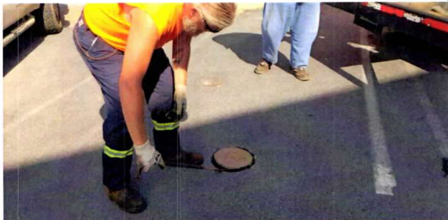
View of Eco First accessing the 1,000-gallon UST. Photo taken from the southeast, facing northwest, on 8/14/2018.
