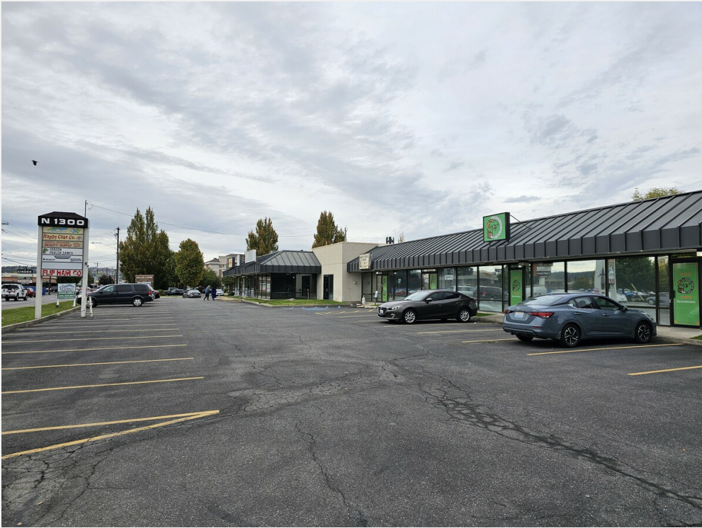
Building South End
