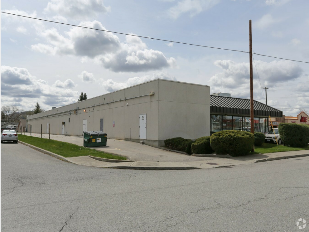
Back of Building
