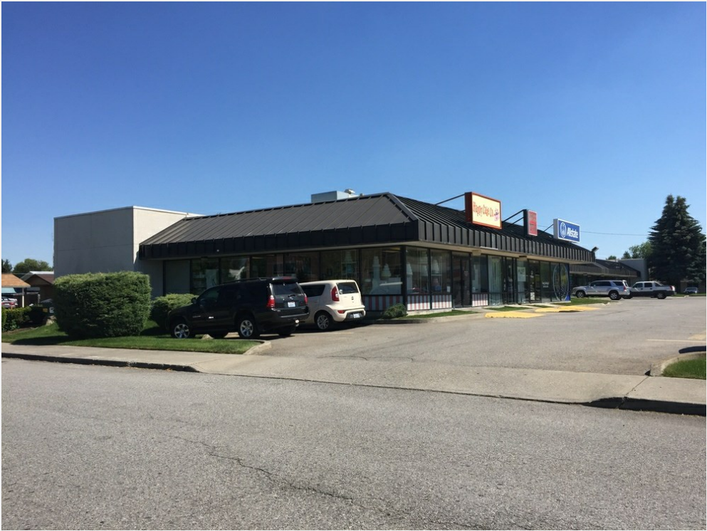
Curb Cut N End
