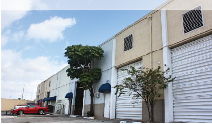
Kelsey Business Center at Park Road
