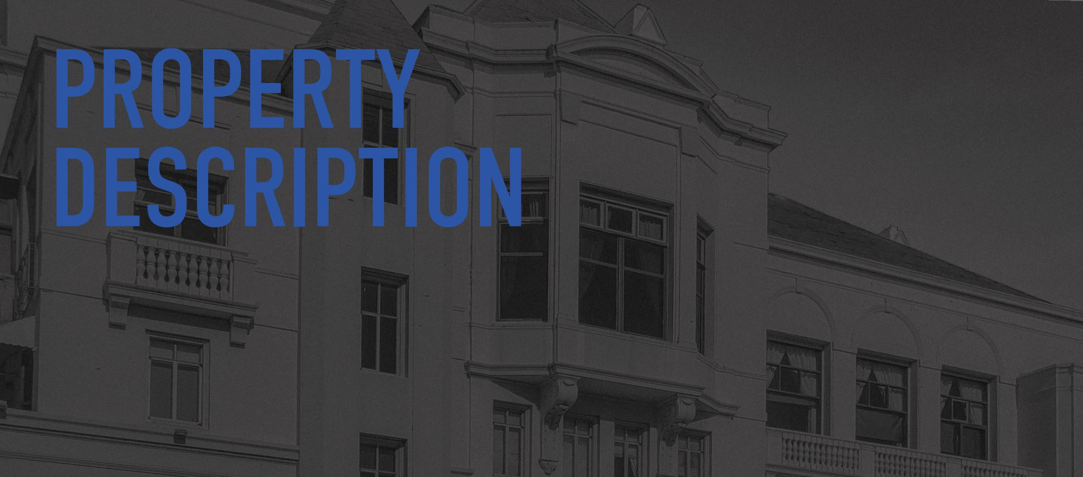
The Property was completed in 1929. It was designed in 1927 by a well known architectural firm of the era, Charles F.B. Roeth & E. Geoffrey Bangs. It is constructed with in-place poured concrete structure with five stories including a full basement and garage level that extends to the rear of the property under a parking deck. The property sits on a reinforced concrete perimeter and pier foundation that has numerous grade beams and reinforced bearing points.
