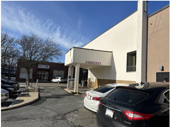
Former Bank Drive-thru
