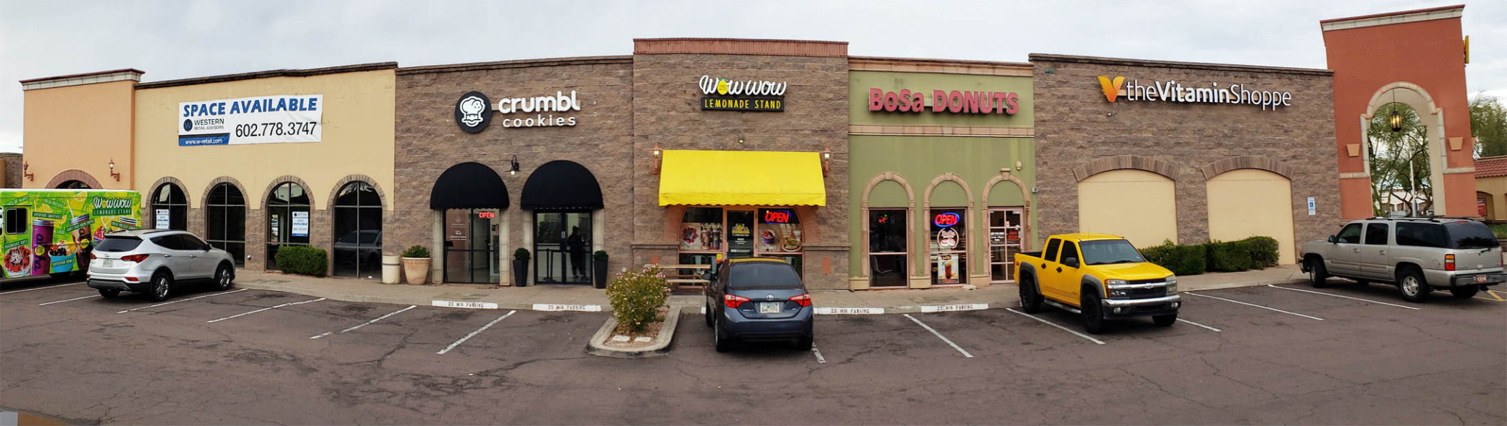
Building G - Side 1
