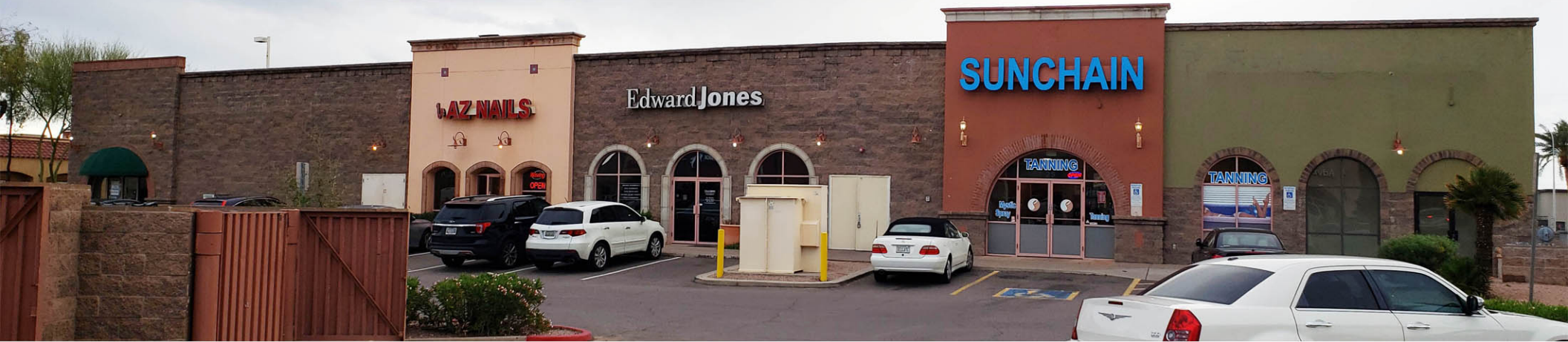
Building G - Side 3
