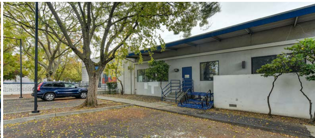
PATIO ON NORTH SIDE OF BUILDING
