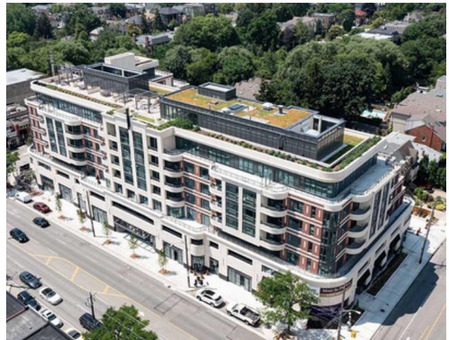
New mid-rise residential on Avenue Road
