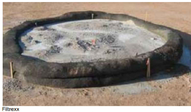
FIGURE 3.18 Typical Compost Sock Washout Installation
