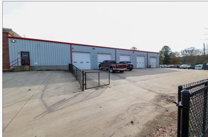
5-Bay Warehouse Fenced Storage Area
