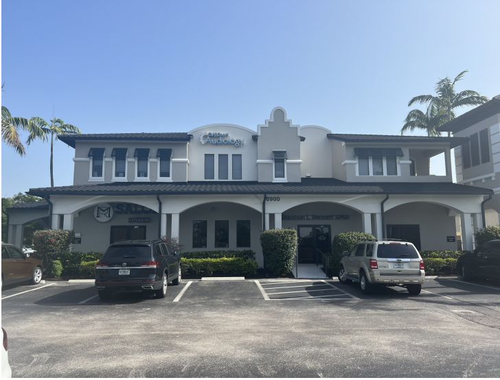
Front of Building
