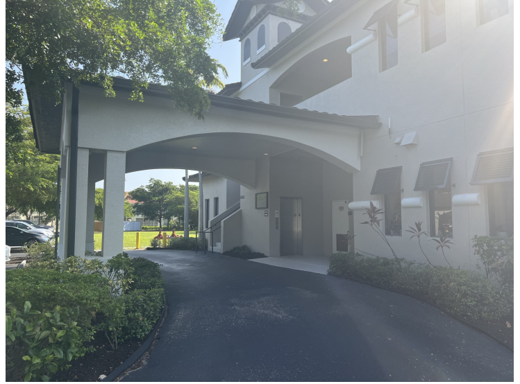
Covered Drop-Off At Stairs and Elevator
