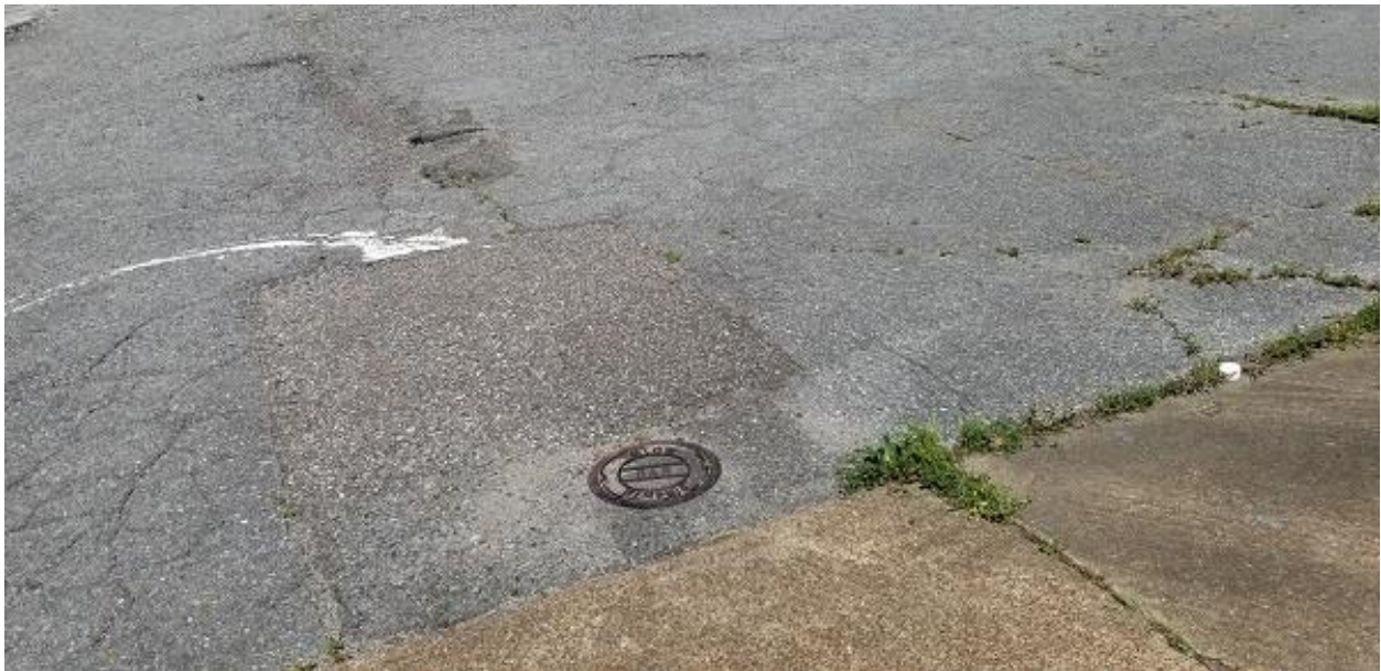
Photo 4: Gas meter cover on south end of property
