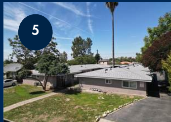
7032 GLASGOW AVENUE SAN BERNARDINO
