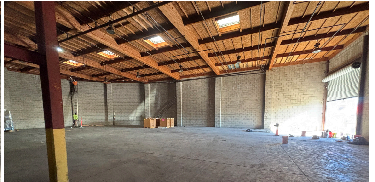
Concrete Block Addition (20' Clear)
