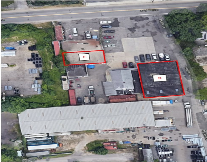
54 Union Ave - Unit Labels
