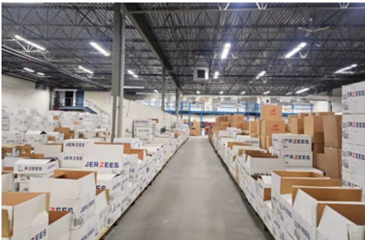
Warehouse 1: Exhaust Fans Throughout
