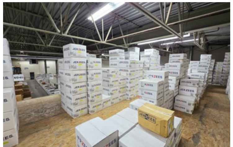
Storage Steel Mezzanine
