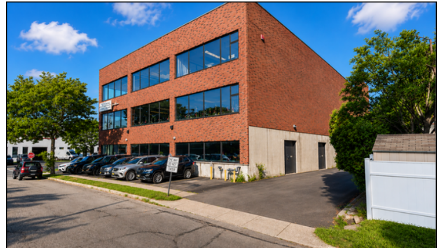
TWO DRIVE-IN DOORS ACCESSIBLE FROM BERKELEY ROAD
