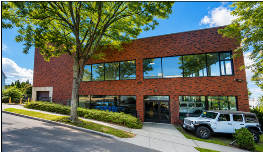
SHOWROOM ENTRANCE & DRIVE-IN DOOR ON MARLBOROUGH TERRACE
