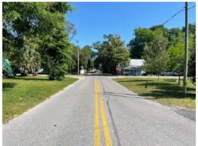
CLYDE STREET FACING NORTH
