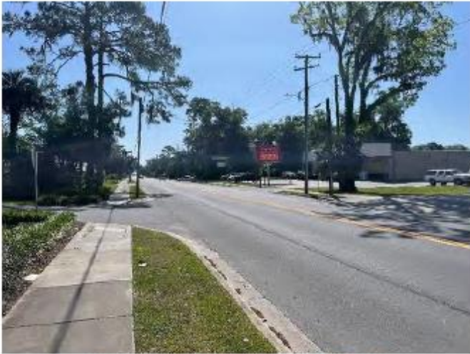
E MAIN STREET FACING EAST
