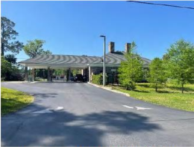
DRIVE-THRU EXIT TO BOXHAM STREET
