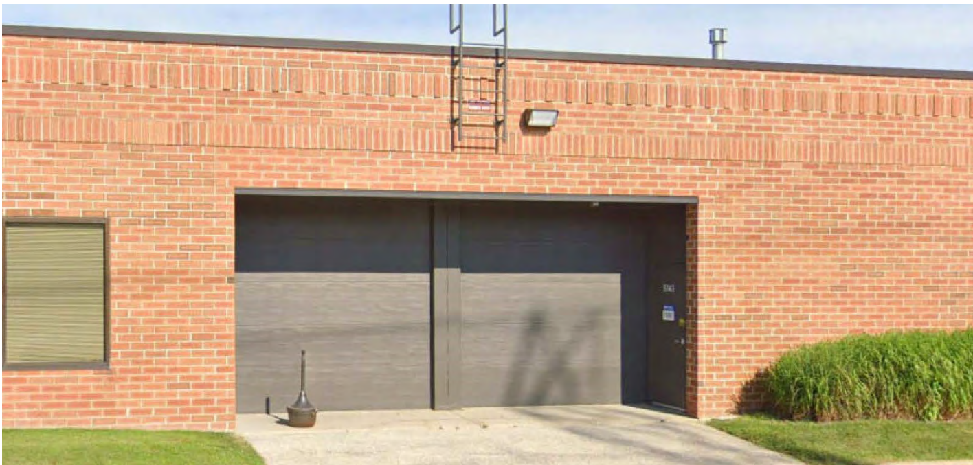
Overhead door and/or dock access potential
