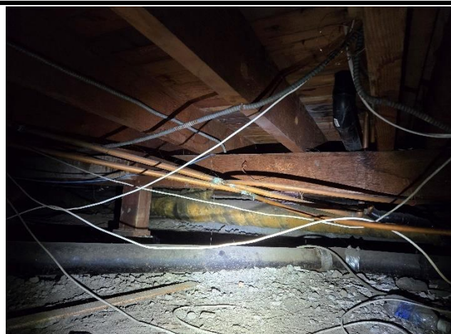
Photo 24 – Typical Crawlspace View
