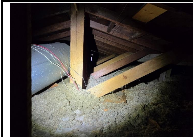
Photo 23 – Typical Attic View
