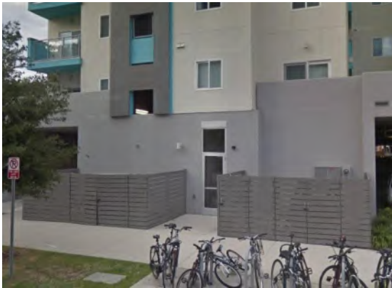
Allowed (utilities screened by fence)
