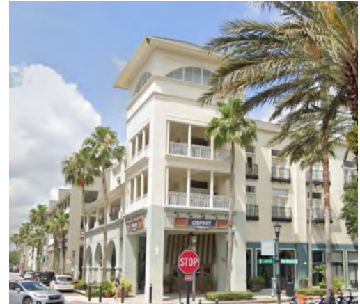
Figure 5 - 15: Small Footprint Tower (top) and Cupola (bottom)
