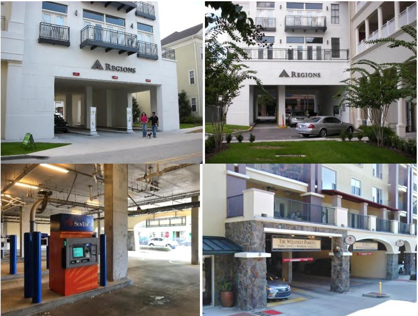
Figure 5 - 36: Interior Drive-Through Facilities
