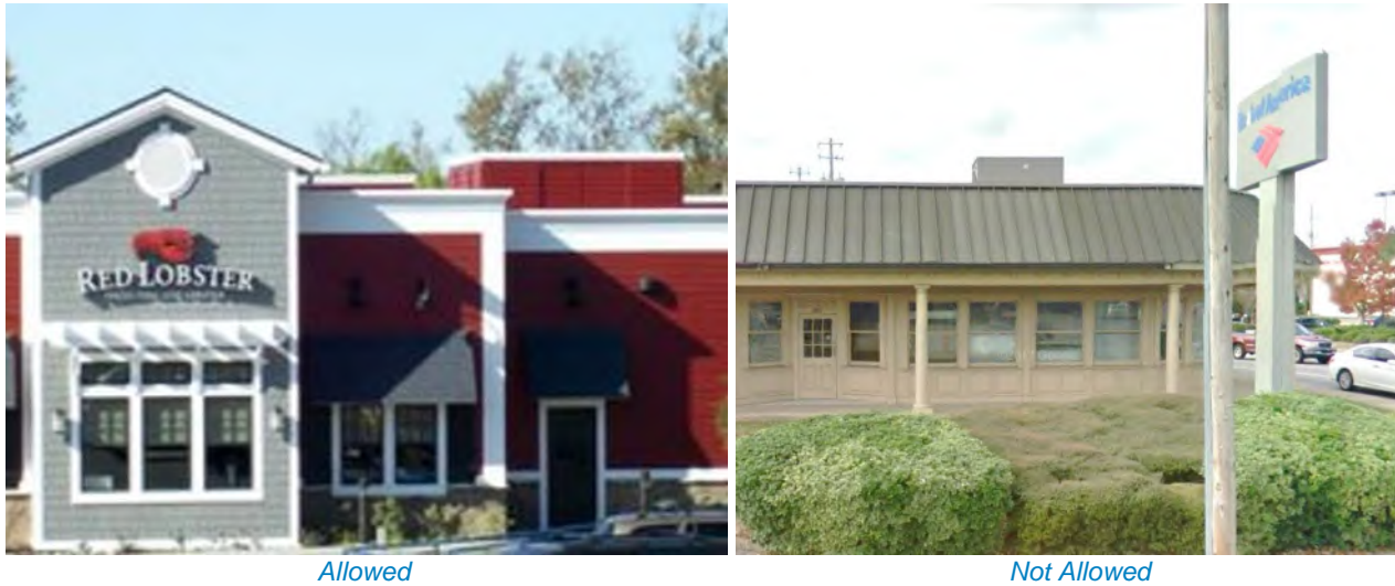
Figure 5 - 32: Rooftop Units Screening
