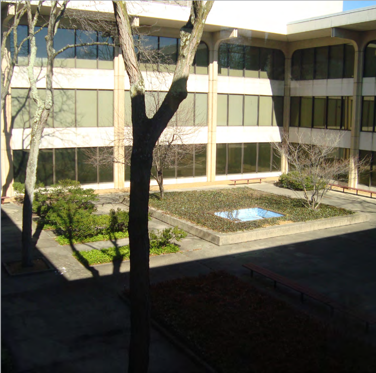
COURTYARD "D" BUILDING
