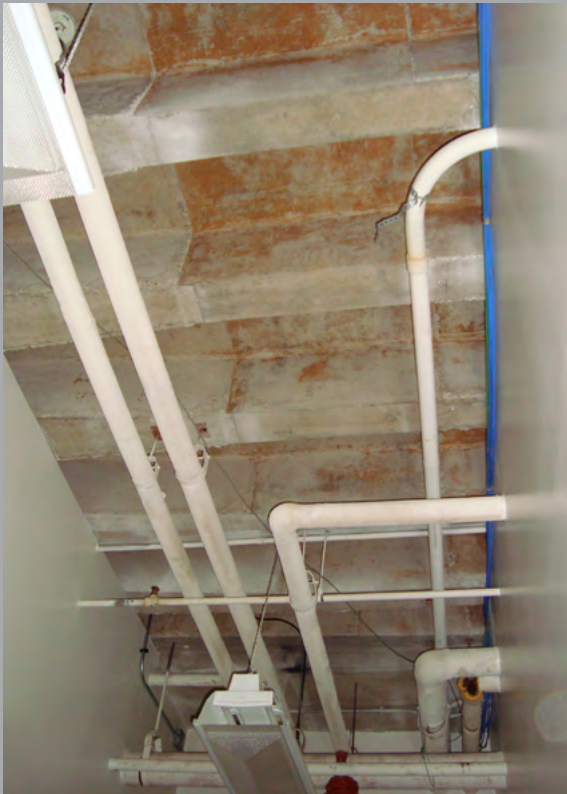
THICK CONCRETE DECKING AND COLUMNS
