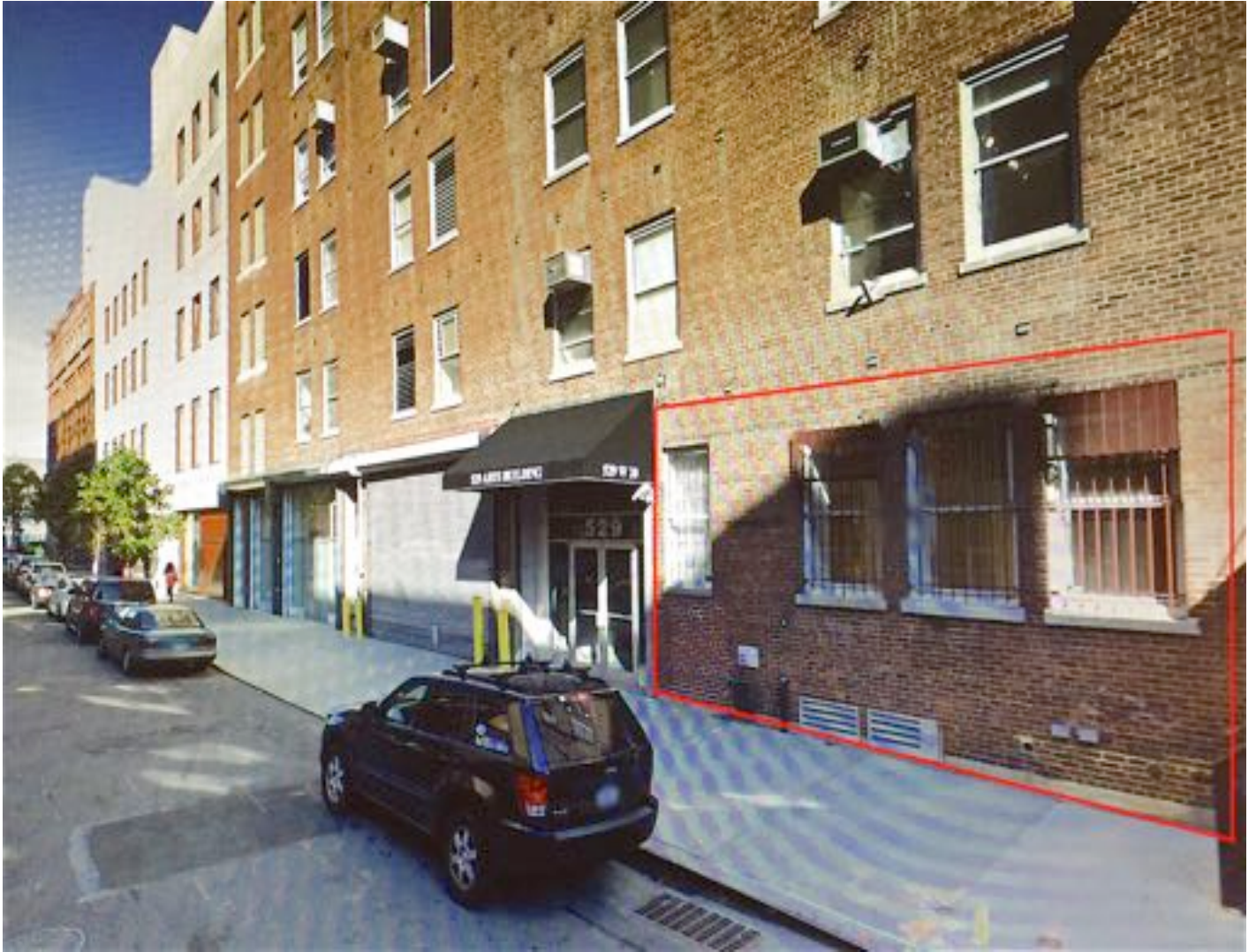
Current facade, 30' frontage
