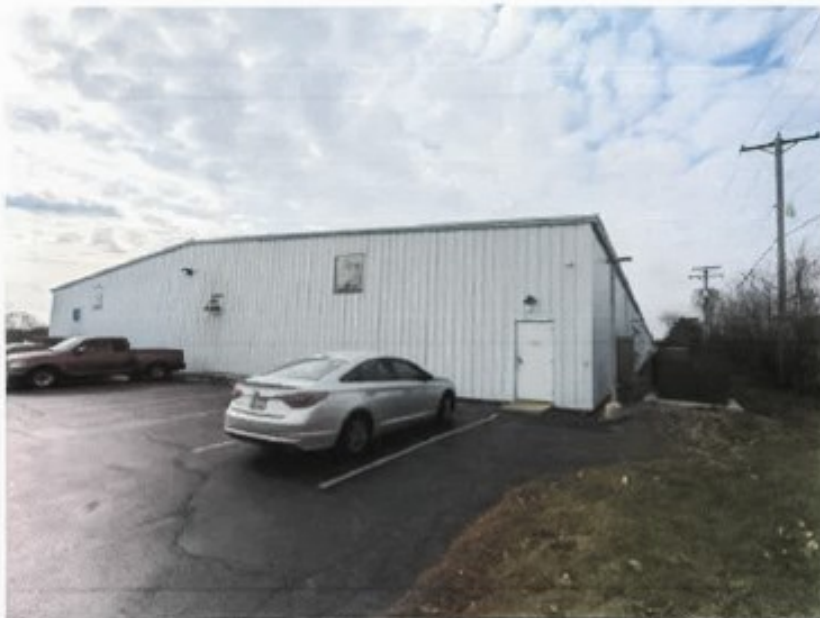
Subject Building Viewing Southwest
