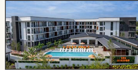
The Station at Alta 302 units (2024)
