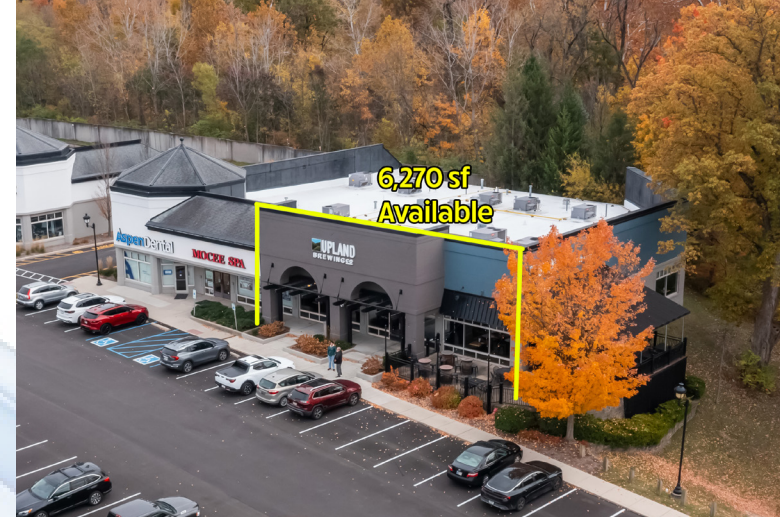
Building D Unit 100 6,270 sf available
