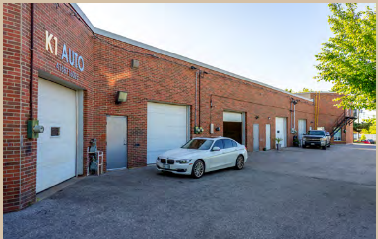
DRIVE IN DOORS
