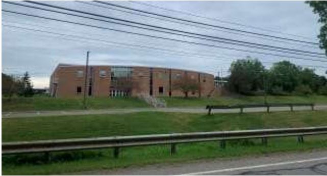
FRONT VIEW FROM STATE HWY 18
