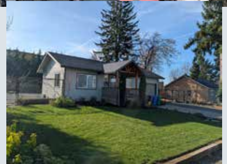
Renovated home used as office
