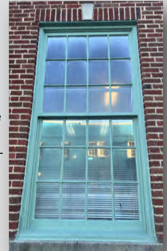
12 over 12 wood window on E. Howell side.
