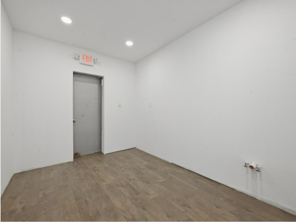
Back Room/ Plumbing
