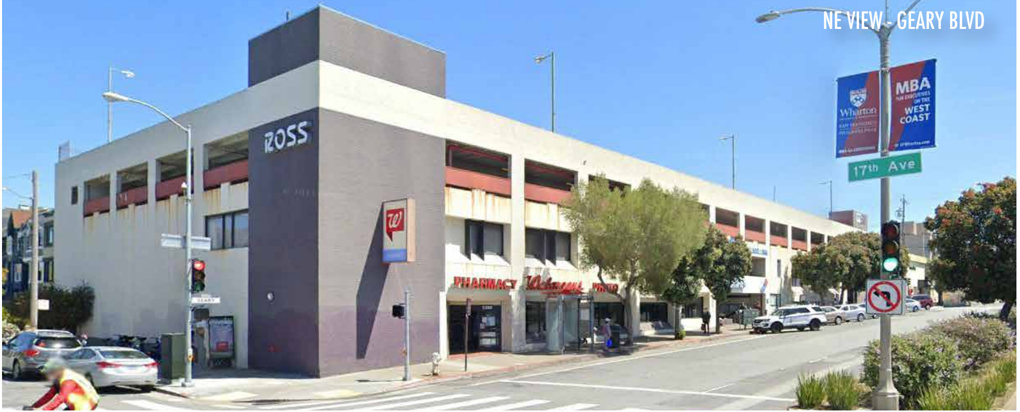
PARKING GARAGE ENTRANCE - 16TH AVE
