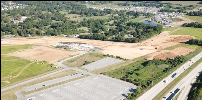
Easton, PA | 500,000 SF Flex | Under Construction
