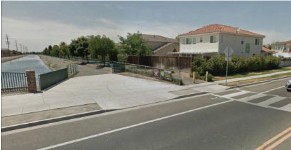
MID Main Canal at Oakdale Road
