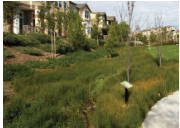
Bioretention areas are shallow, landscaped areas that receive and treat stormwater.
