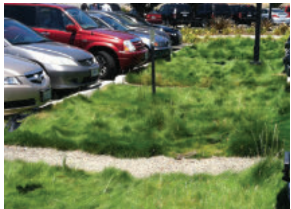
Vegetated swales are shallow stormwater conveyance channels with vegetation covering the side slopes and bottom.
