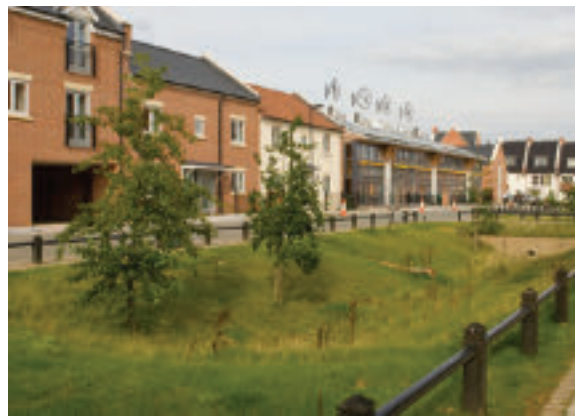
Basins that are thoughtfully designed and planted can manage stormwater from a larger area, while still offering aesthetic appeal.
