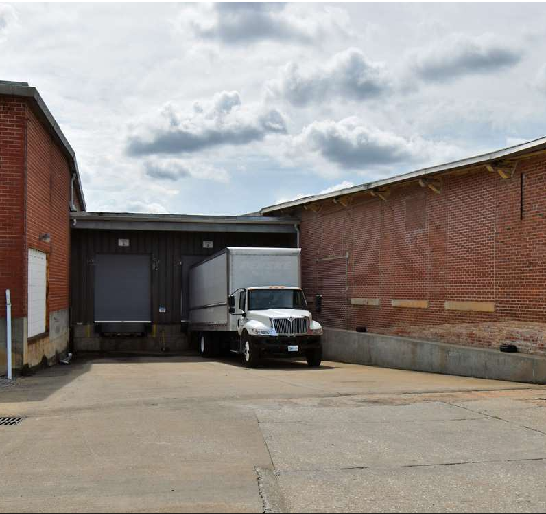
River Mill 6 loading docks
